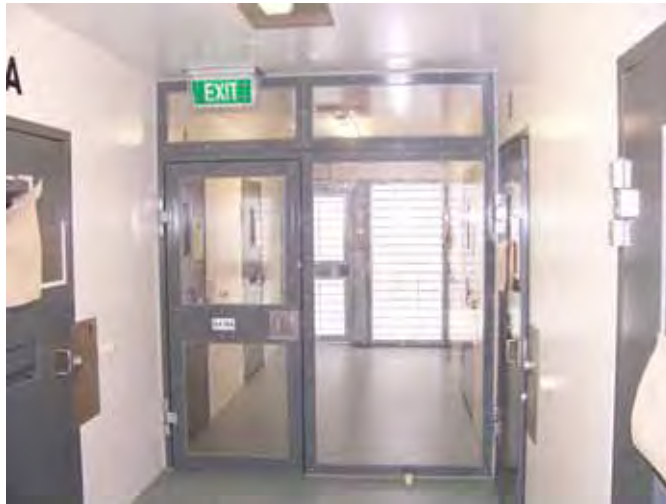
Cells at the eastern end of the unit and entrance to smaller yard.
